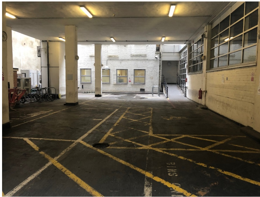
3.5 Image 6 - Rear Servicing and Parking Area (Undercroft)
