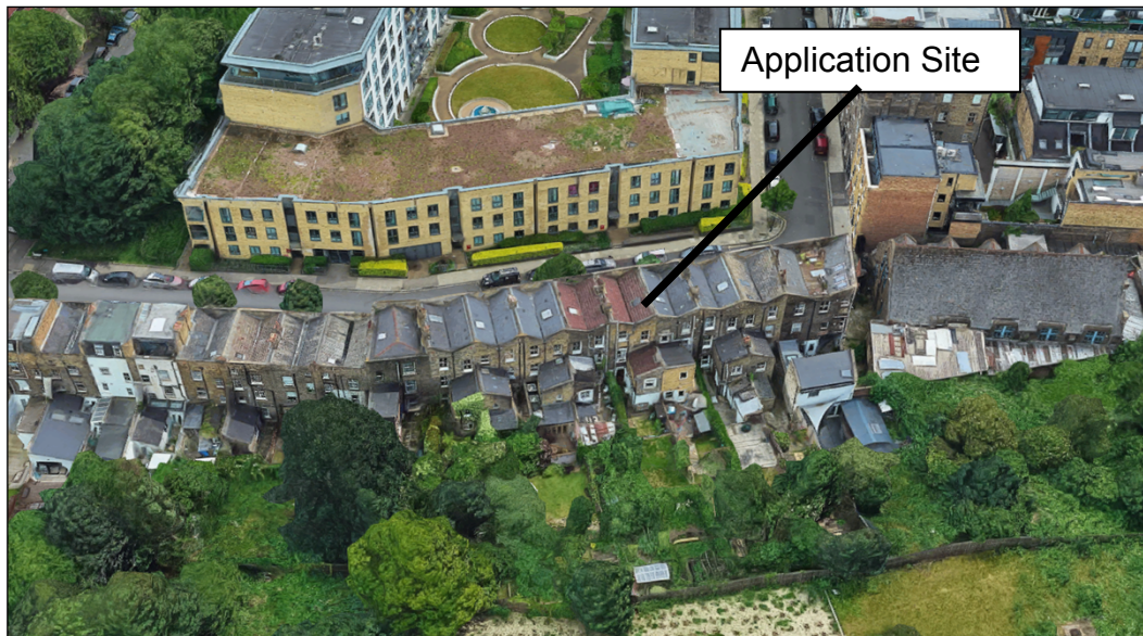
Figure 2: View of rear elevation
