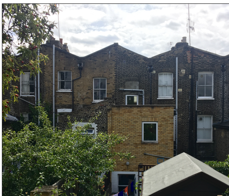
Figure 5: View of rear elevation of Nos. 92 (left) and 94 (right) Gifford Street
