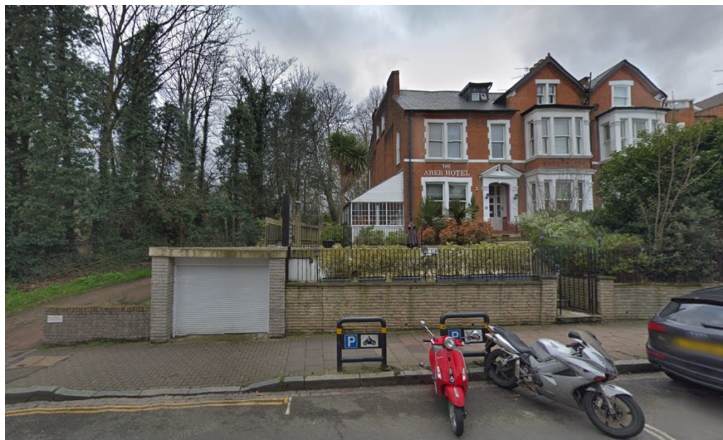
Image 2: Photograph from street level showing the front elevation
